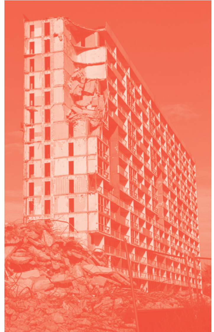
Demolition of the Balzac tower, symbolic building of the «Cité des 4000» at La Courneuve, France in 2011 © Diego BIS / Flickr.
