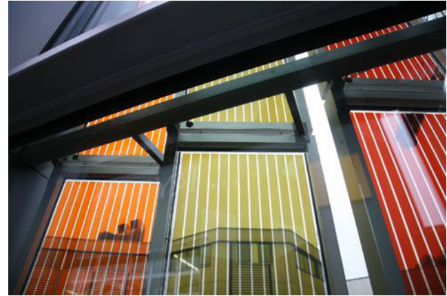
Fig 9. Swisstech convention center , façade made by Solaronix in 2014
